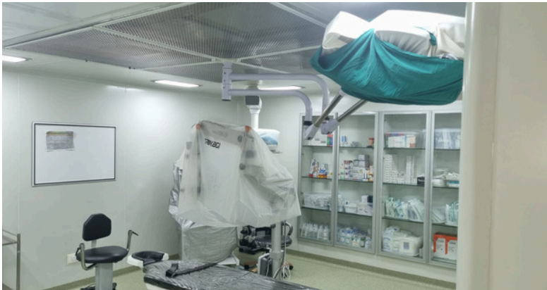
OT upgradation in progress
